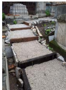
Steps to hold back soil and deal with level changes
