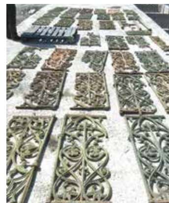
Dismantled Cast Iron Balcony to be restored and replaced at St Bernard's School
